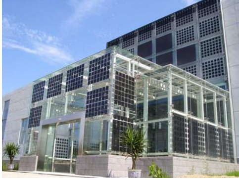
Figure 5-5: BIPV window
