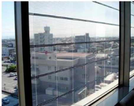
Figure 5-9: BIPV Window
