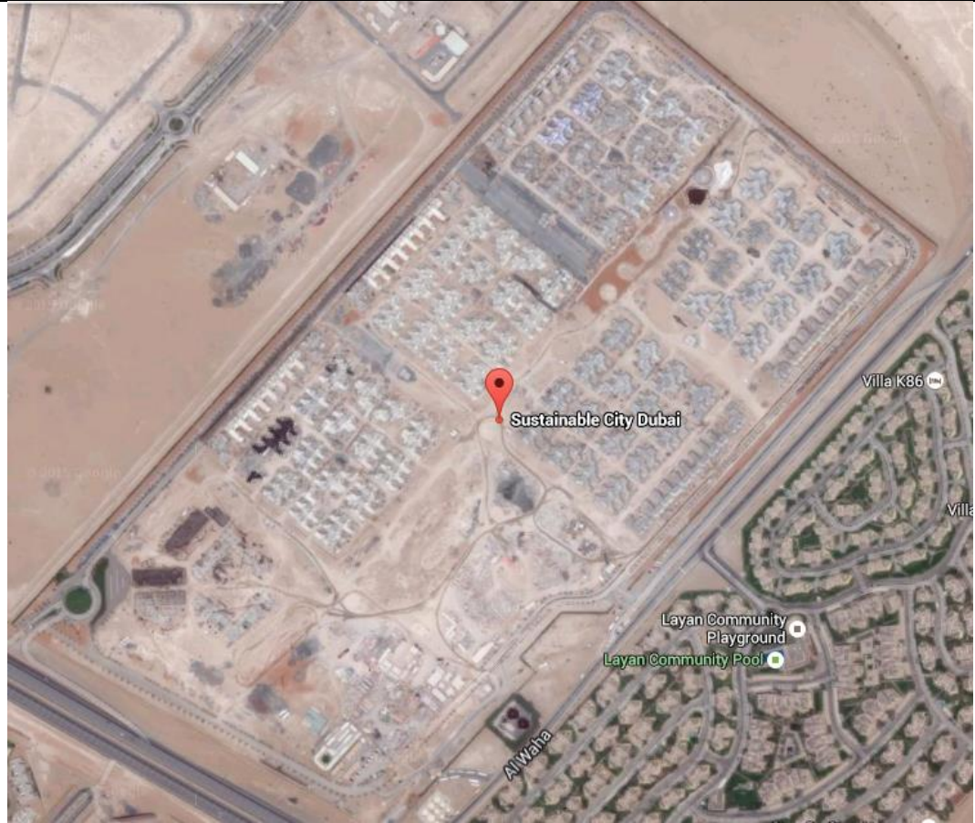
Figure 5: The location of the TSC in Dubai and the most recent satellite image of the TSC progress in construction (July 2015)
