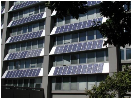
Figure 5-3: BIPV Solar Shade
