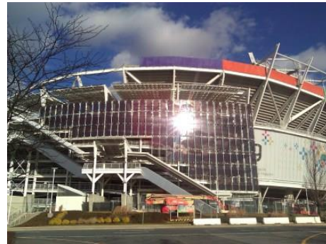
Figure 5-4: BIPV Rain Screen
