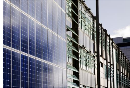
Figure 5-12: BIPV Façade
